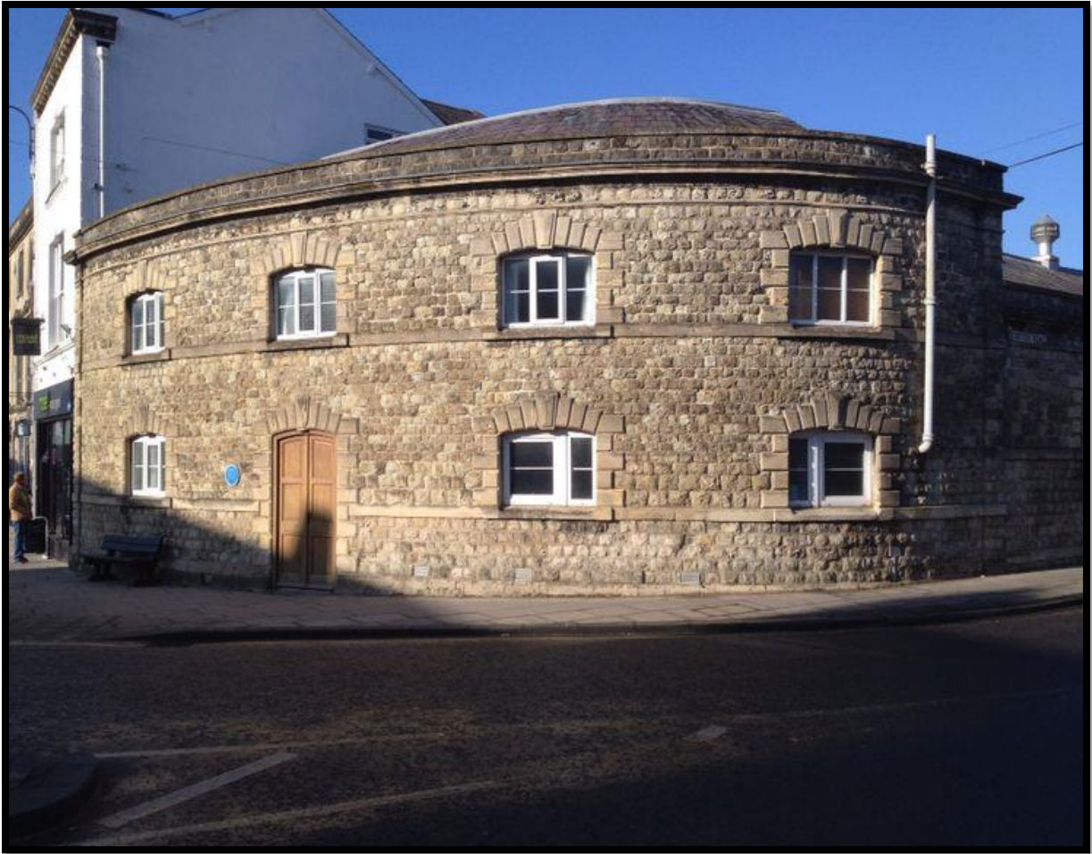
Above: Masonic Lodge at Warminster
