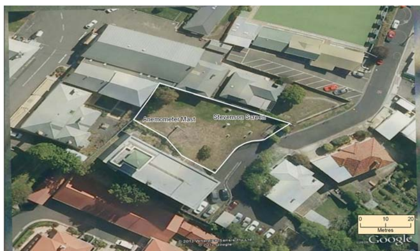
Figure 38. Battery Point (Hobart) Ellerslie Rd. meteorological observing site illustrating the urban setting surrounding the anemometer mast.
