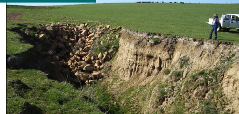
Head cut in top of gully, rock used to slow erosion. Photo Rick James
