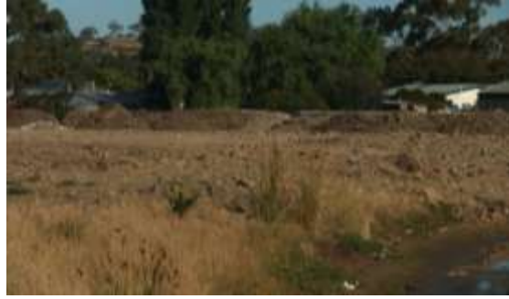
Fill to raise land levels
