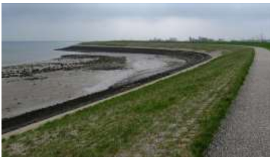
Dyke with coastal road, Holland
